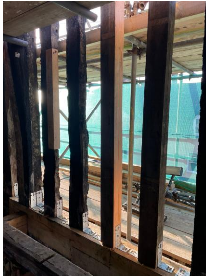
Studwork wall mixing new and still structurally sound charred timbers
