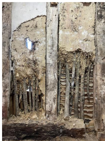
Wattle and daub panels showing natural wood
